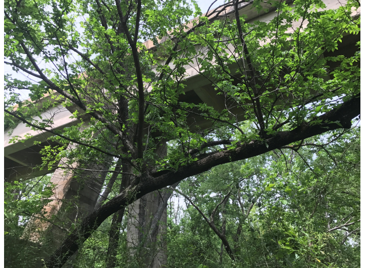
The Interurban Bridge along Jefferson Avenue.
